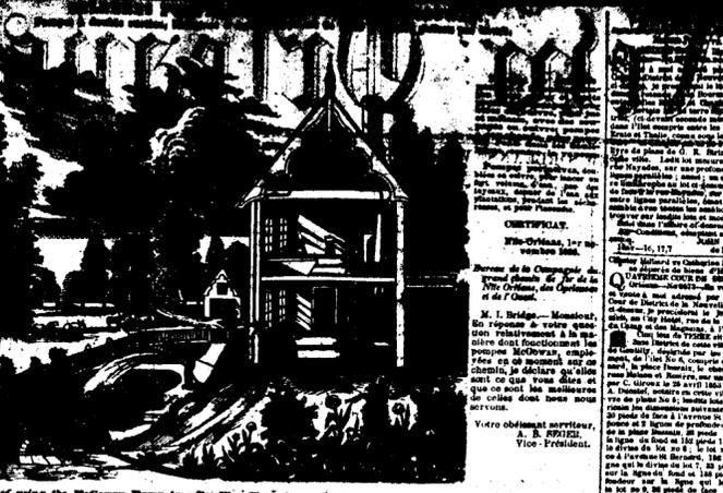
Method of using the American Pump in a building to supply steam, and protect the building from fire.
